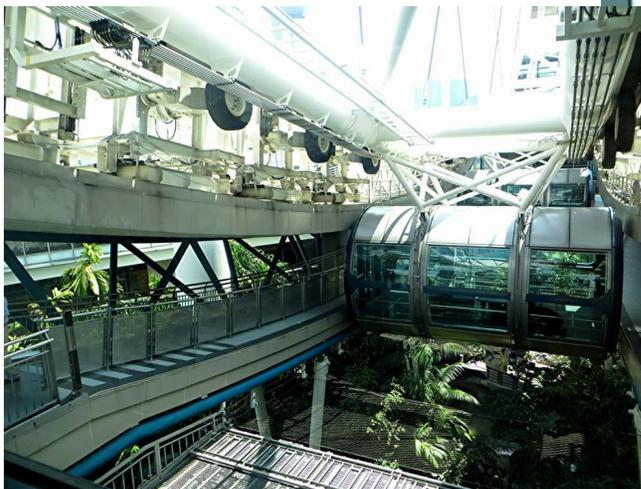
rubber tires in the base building that contact the massive outer steel ring of the wheel, as shown in this picture. A similar set of tires contact the upper surface of the outer ring to keep it from tipping over in a high wind.
